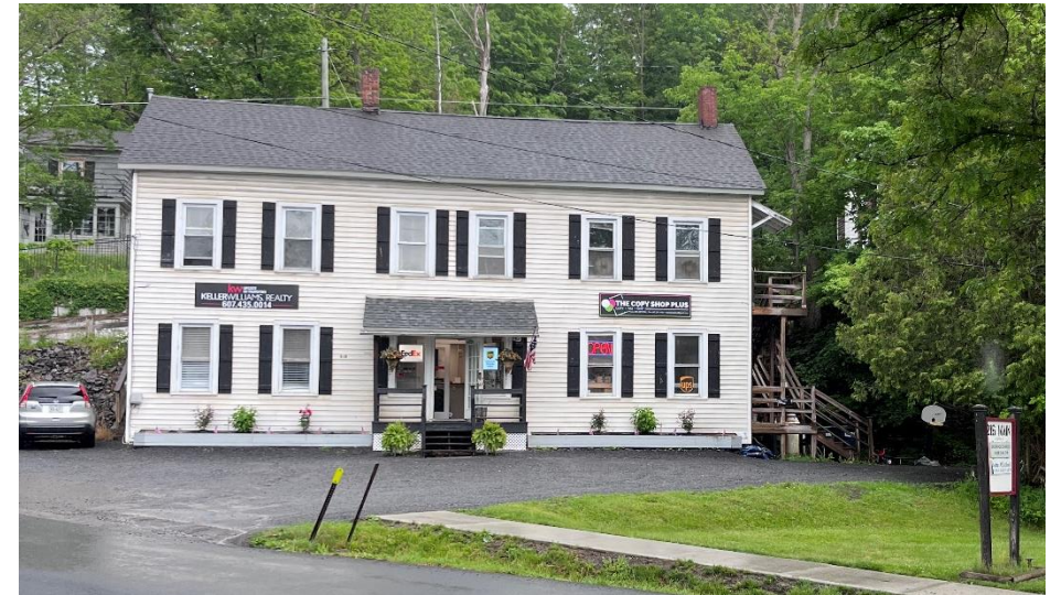
Downtown Row Type (top) Converted Residence (bottom)
