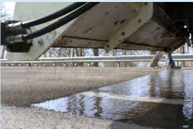
Automated application of HFST. Source: FHWA
